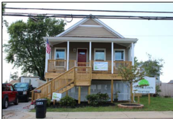
The new Hoffman residence, which was rebuilt after Hurricane Sandy, features two bathrooms outfitted with American Standard Cadet PRO high efficiency toilets, Colony Soft faucets and Aqualyn lavatories, all donated by the New Jersey-headquartered plumbing manufacturer.
